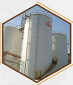
Bulk oil storage tanks
